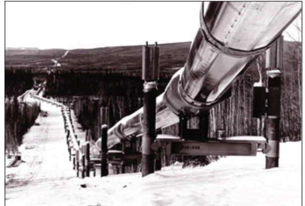
Civil engineers helped design and construct the 800-mile Alyeska Pipeline, shown near Livengood in this 1959 Alyeska photo. The pipeline crosses three mountain ranges and more than 800 rivers and streams. Soil that shifted due to permafrost was just one problem engineers had to solve during construction.
