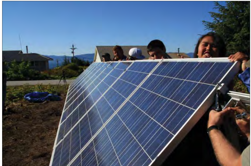
Angoon residents install a solar power panel on a home as part of the Sustain Angoon Project. Photo courtesy of Central Council, Tlingit and Haida Tribes of Alaska.
